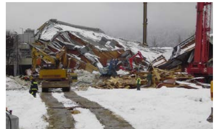
Figure 2. Collapsed roof due to heavy snow fall (photo by Norbert Gebbeken)
