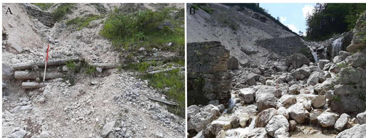
Figure 32. Completely destroyed torrent control measures that provide no protective function. Location: Kranjska Gora. (Photo: Domen Oven).
