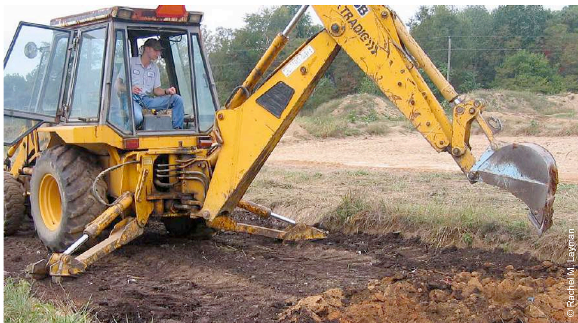
Photo 66. Compost application. During the compost application and backhoe subsoiling, the operator must scoop a bucket of soil with compost on the top, lift it several feet in the air, and drop it. This breaks up the compacted soils into large clods and creates veins of compost down
