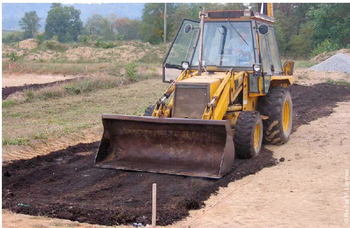
Photo 65. In the profile rebuilding technique employed in the Virginia case study in 2007, the compost is spread 4 inches (10 cm) deep over the soil surface
